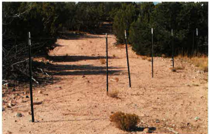
Image III-4: Five-Strand Barbless Wire Fence along the west side of Camino de los Montoyas.
