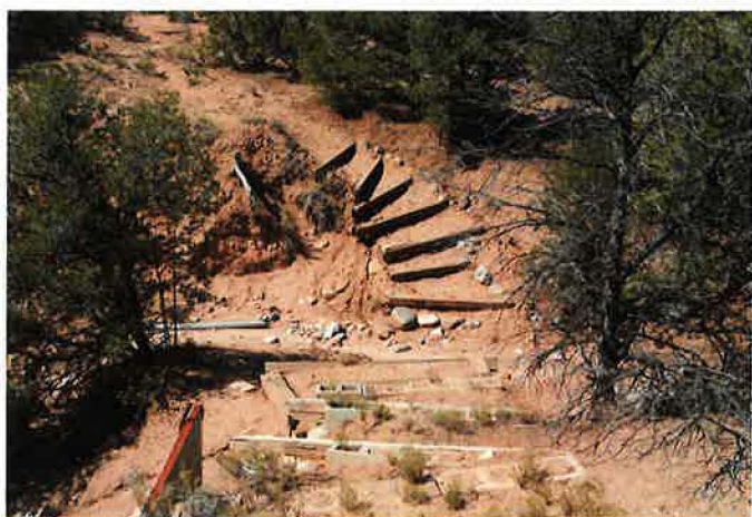
Image I-13: Dilapidated steps at the old archery range are washed by a gully.
