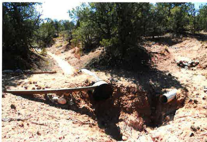
Image I-11: Walkways with old culverts at the old archery range drain into a highly eroded low point.
