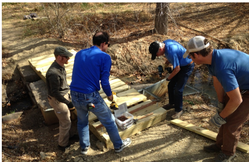
Figure 13 Santa Fe Fat Tire Society members install a bridge to complete the Cerro Gordo Trailhead Connector
