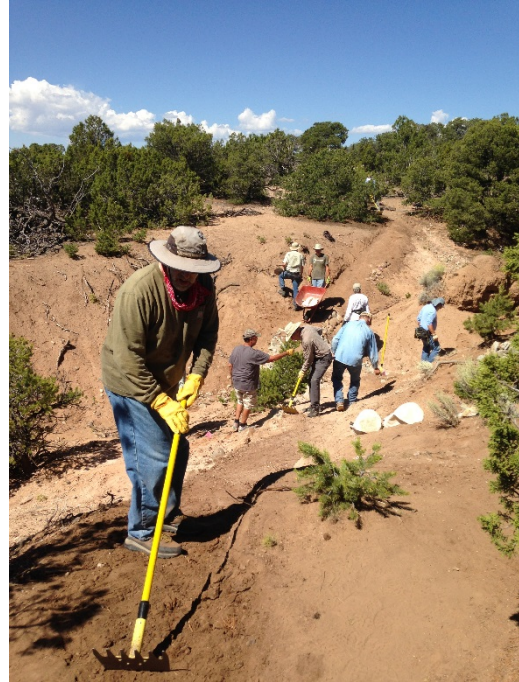
Figure 8 Volunteers building the Arbolitos Trail
