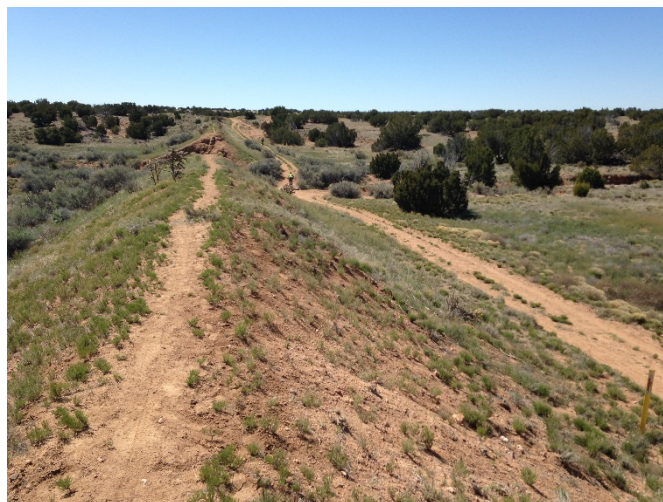
Figure 11 NM Central Railroad on south side of Rancho Viejo
