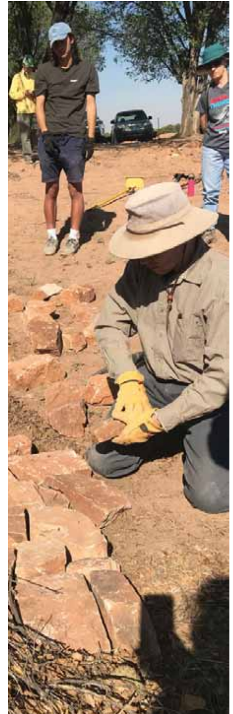
Above: Building a one rock dam on The Conservation Homestead
