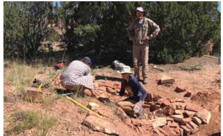
Above: constructing a Zuni bowl on the Conservation Homestead
