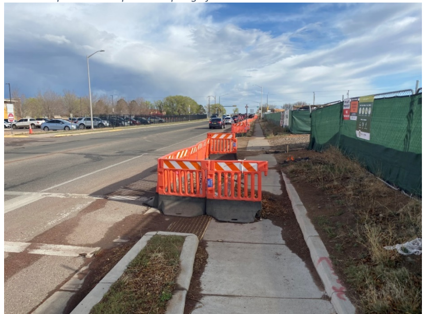
Figure 48 Engineering concerns also include maintenance and operations. For the sake of a single construction driveway crossing, this otherwise viable 500-foot stretch of sidewalk along South Meadows Ave was closed for two school years (2022/23 and 2023/24), preventing access from the north to Sweeney ES's school crossing for the duration of a commercial development construction project. The allegedly safer alternative that prospective walkers were directed to was to cross South Meadows at Airport Rd., one of Santa Fe's "top ten" locations of motor vehicle crashes, a fact that the SFSRTS Coordinator shared in discussion with the City Land Use Department on this matter.
