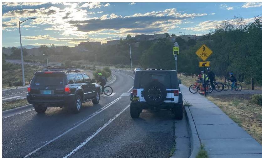
Figure 59 Bump-outs are recommended on Jaguar Dr. to eliminate screening by parked cars at the Tierra Contenta Trail crossing, which is used each Tuesday by the bike train to Nina Otero CS.
